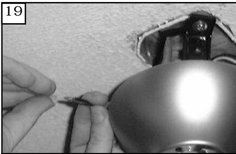
19 Make wire connections to power source using wire nuts provided. Make sure that no filaments are outside of the wirenut. After making the wire connections, the wires should be spread apart with the grounded conductor and the equipment-grounding conductor on one side of the outlet box and ungrounded conductor on the other side of the outlet box.
